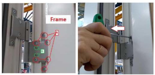
b) Use Allen Key 3mm in order to make horizontal adjustment, please rotate the screws marked with letter B as above
