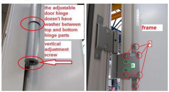
The green marked hinges on the top diagram including the vertical adjustment screw (+ /- 2mm) as shown on the left picture above. The hinges can be also adjusted in horizontal direction with using of screws marked with letter **B** on the right picture above.
